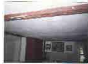
Plaster & beam ceiling in the keeper room
