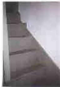
Stairs to second level
