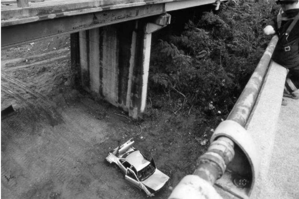
A fall from this height is readily analyzed
